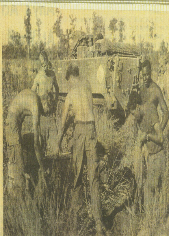
SAND BAGGING - Members of the mortar platoon of Triple Deuce fill sand bags as they build a blast wall for their 81mm mortar track.
